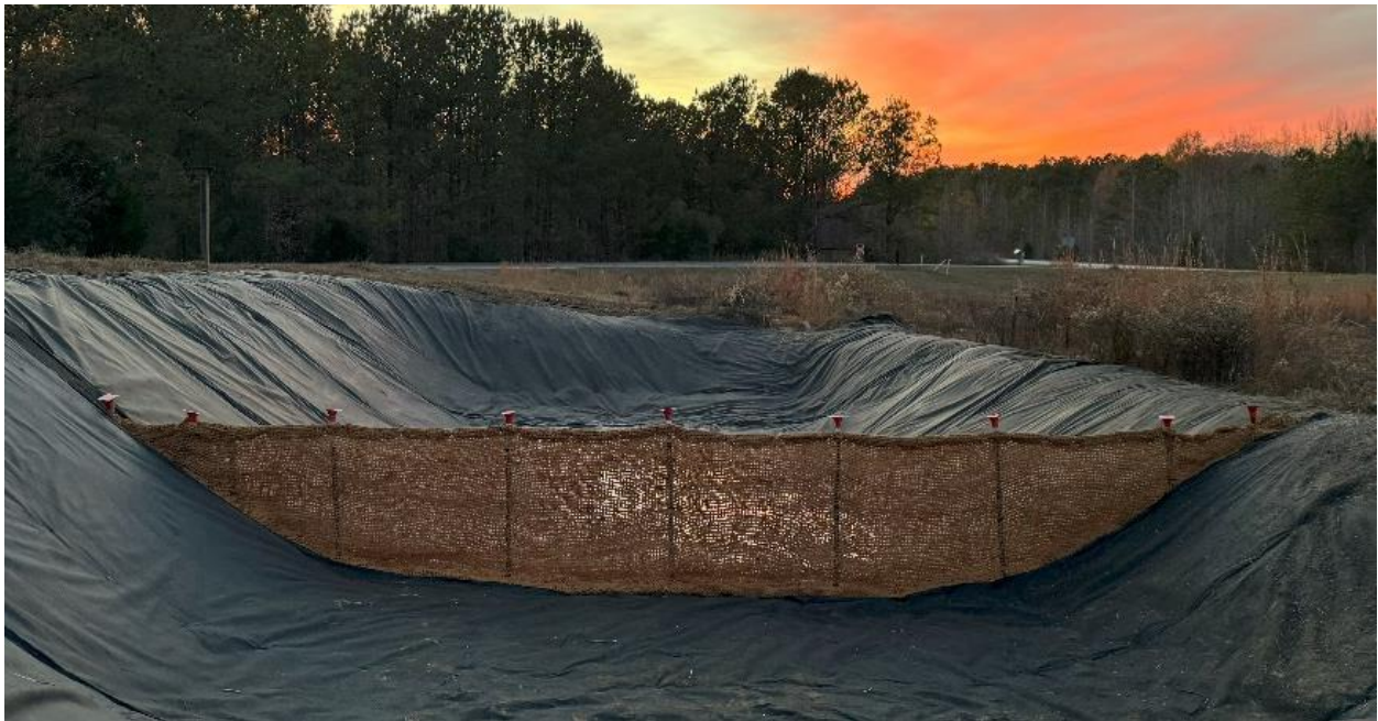
Figure 5.4 Field-Scale Baffle Design.
