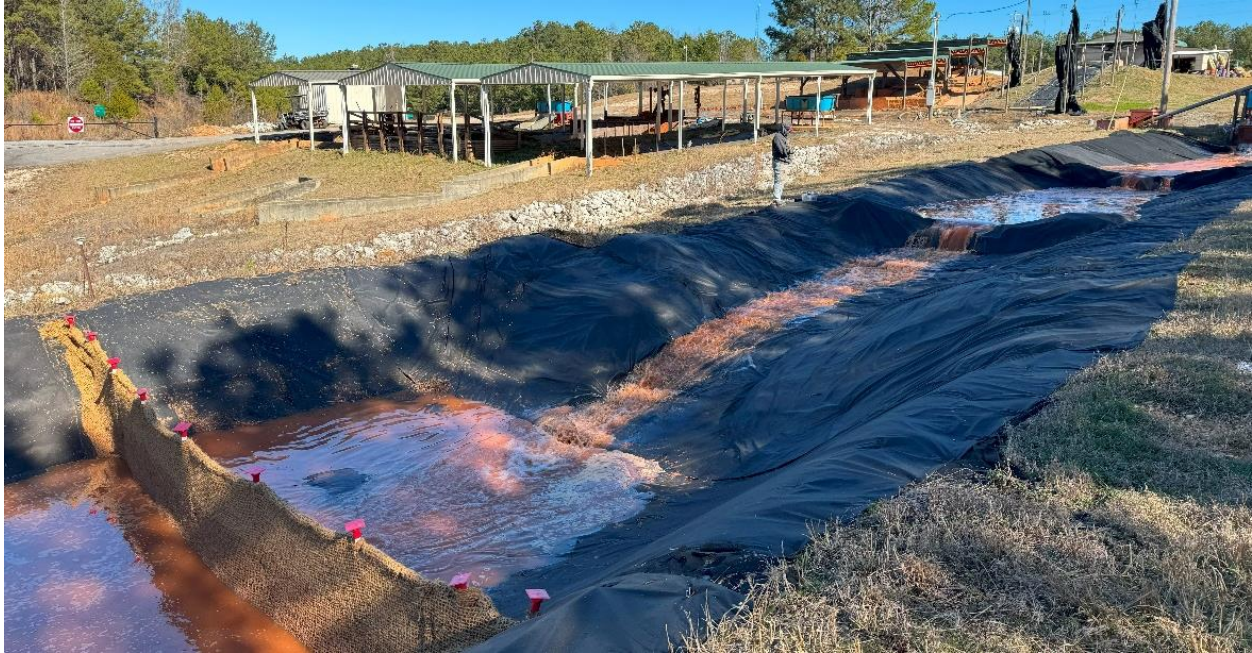
Figure 5.2 Field-Scale Basin Inflow Channel.
