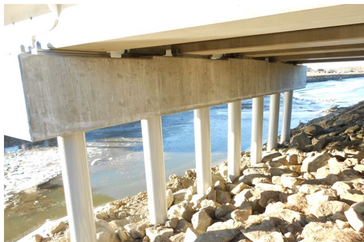
Figure 1-2: Steel pipe piles for bridge substructures (Kappes et al. 2016)
