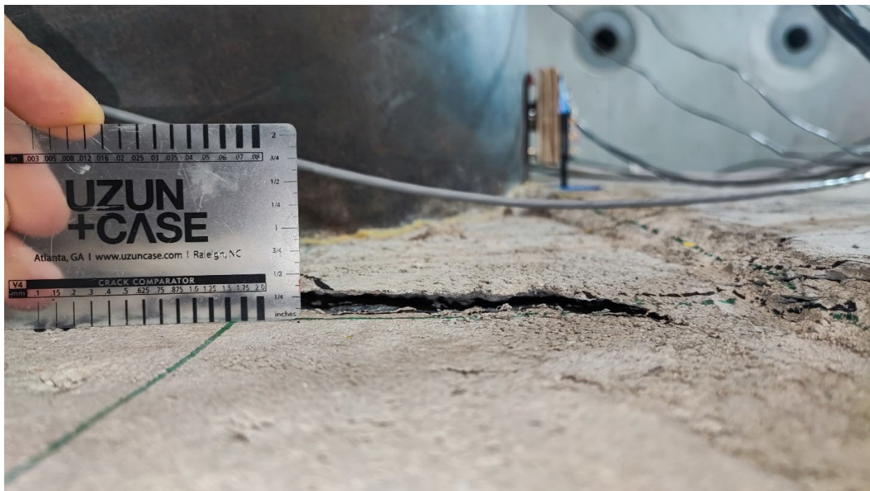
Figure 5-35: Concrete spalling for straight-bar specimen
