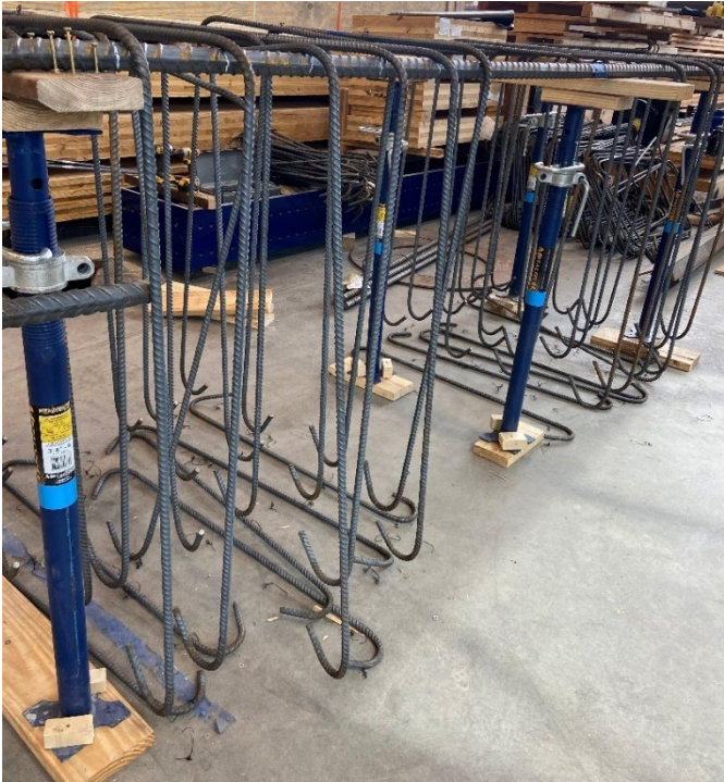
Figure 3-34: Structure to support the reinforcing cage
