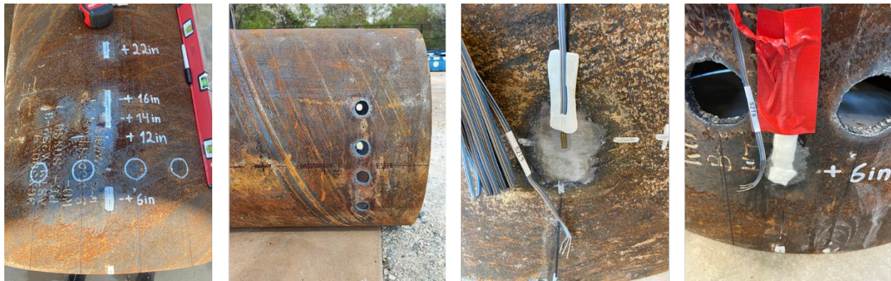
Figure 3-39: Steel pipe pile preparation
