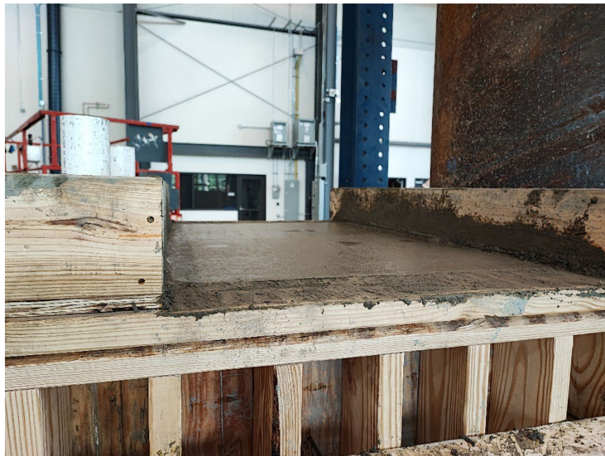
Figure 3-45: Smoothed bent cap surface
