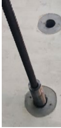
Figure 4-5: Dywidag bar and sleeve
