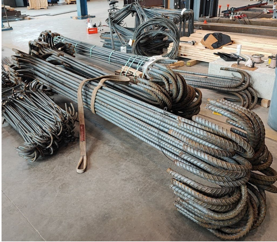
Figure 3-26: Reinforcing bars used for specimen fabrication
