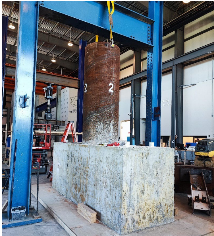
Figure 3-46: Specimen after form removal
