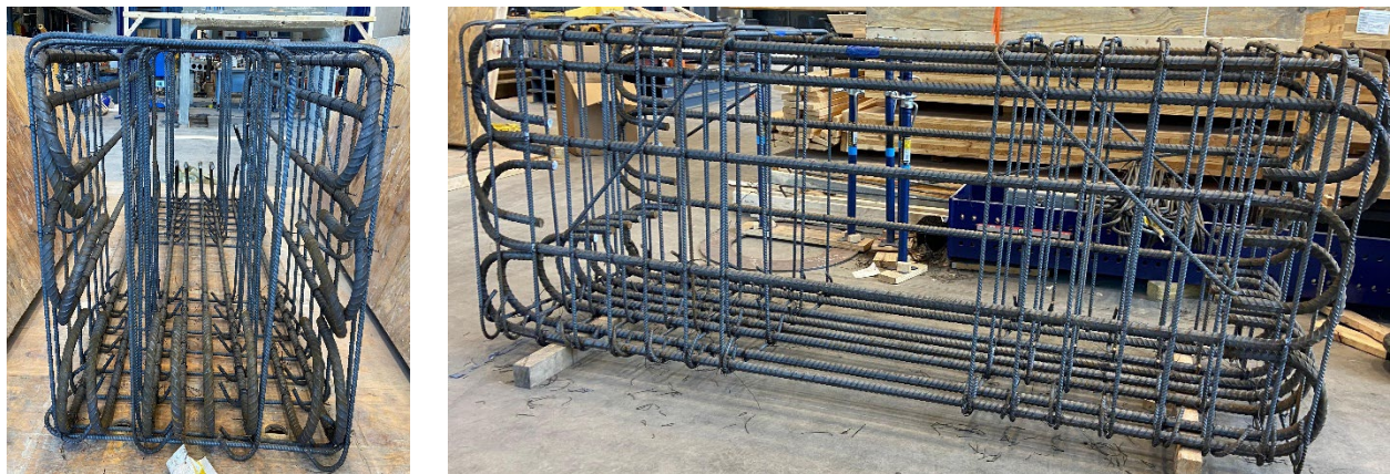
Figure 3-35: Side views of bent cap reinforcing steel cage
