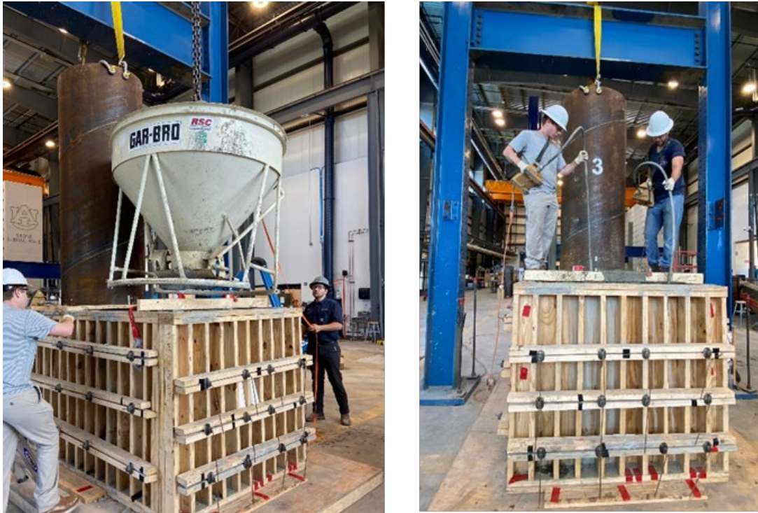
Figure 3-43: Concrete placement process
