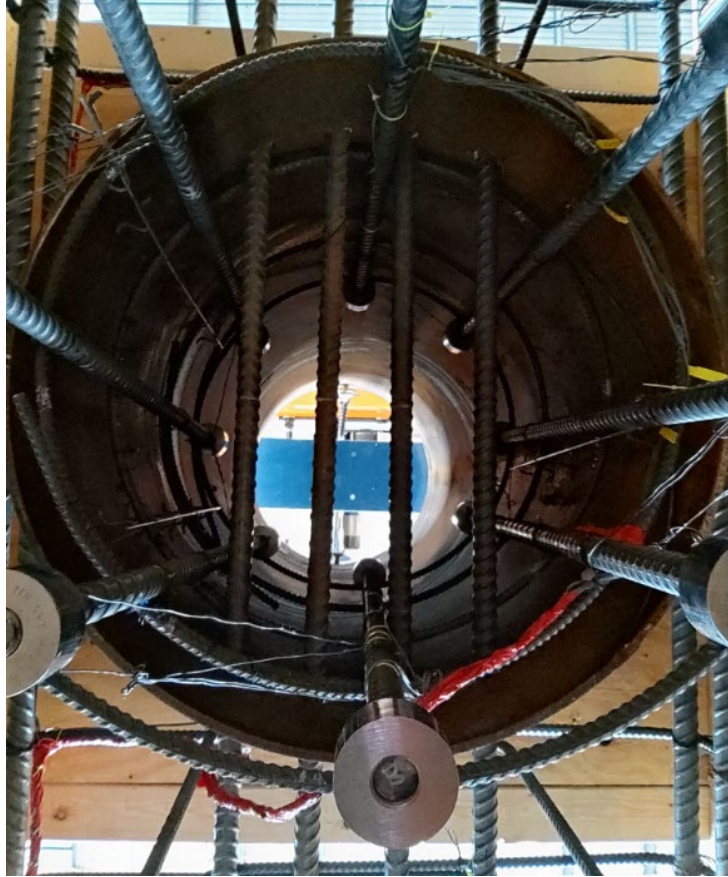
Figure 3-40: Final connection assemblage
