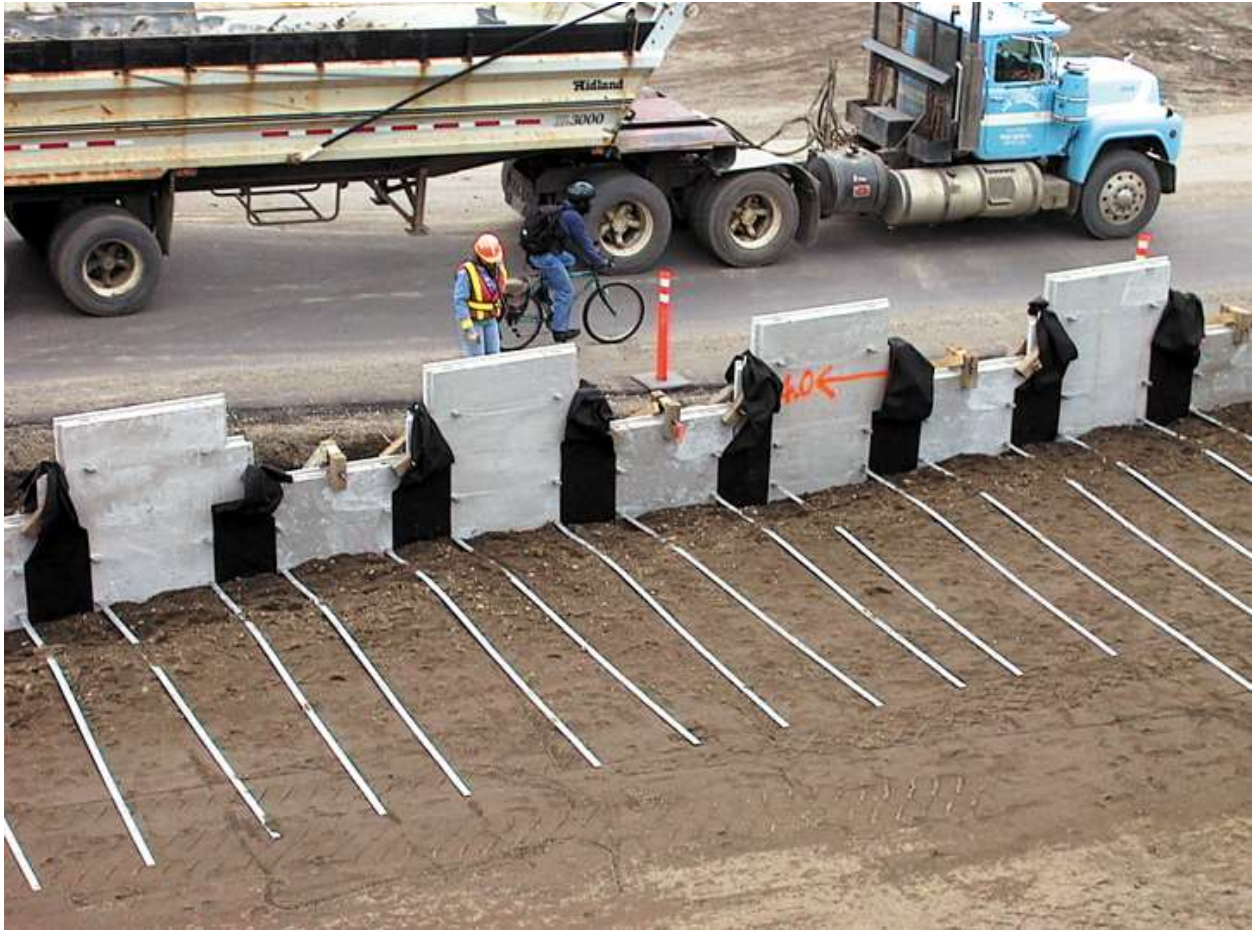
Figure 2: A concrete panel faced, steel strip reinforced structure under construction (Reinforced Earth Company 2008)
