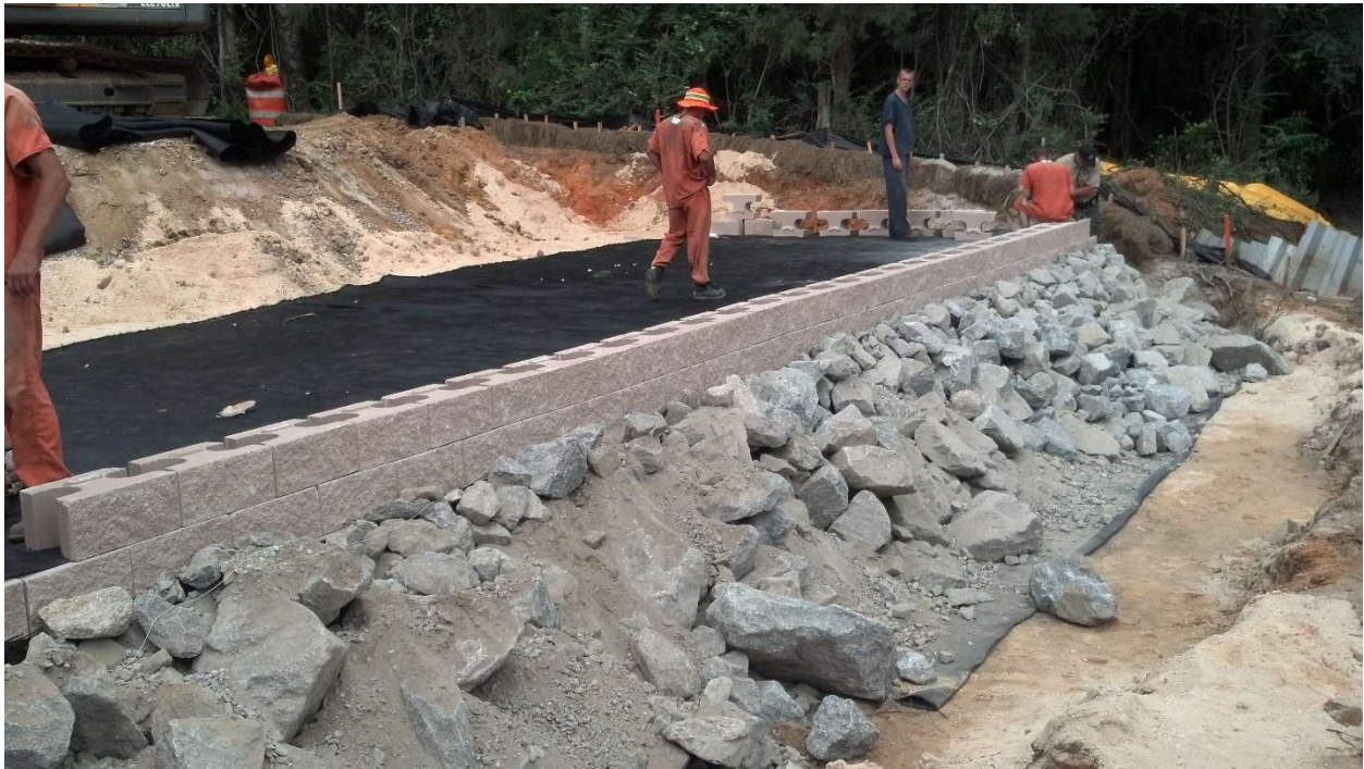
Figure 6: Geotextile sheet reinforcement being used on a GRS-IBS abutment in Escambia County, Florida
