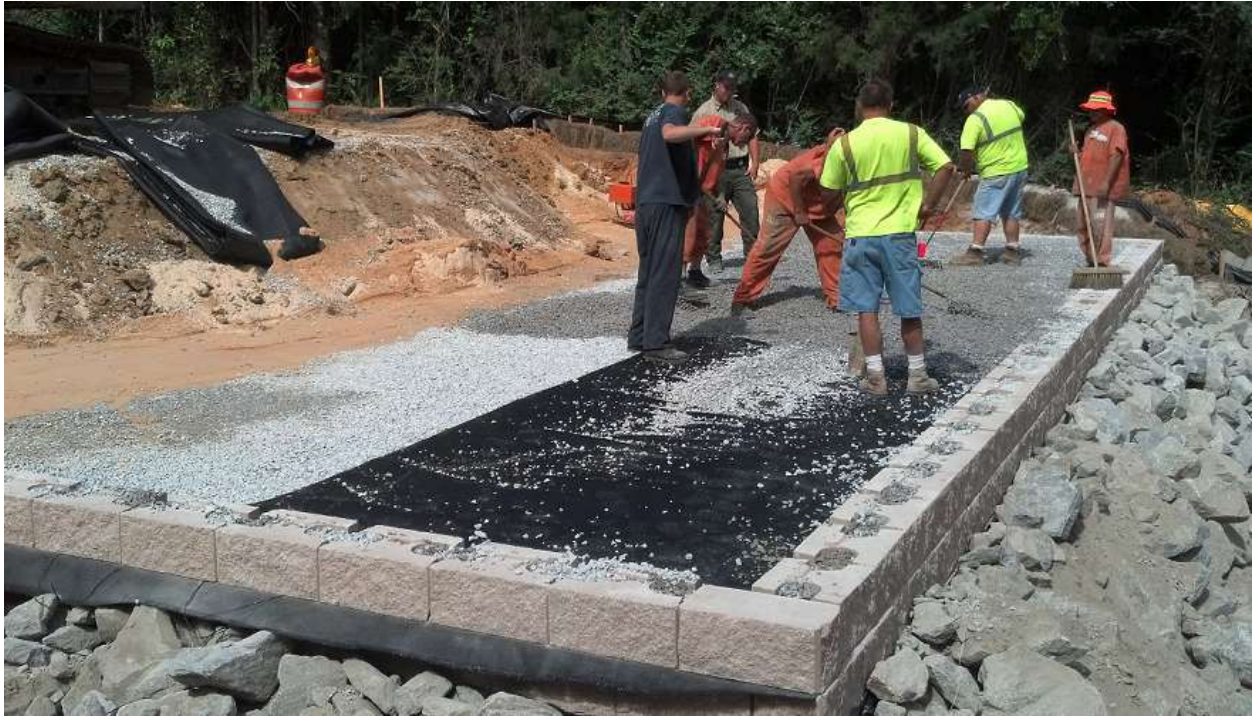
Figure 11: GRS-IBS abutment under construction in Escambia County, FL
