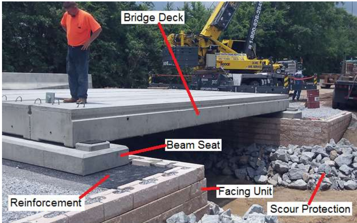
Figure 12: Two GRS-IBS abutments constructed in Escambia County, FL with precast prestressed concrete bridge decking in place, before placement of integration zone soils
