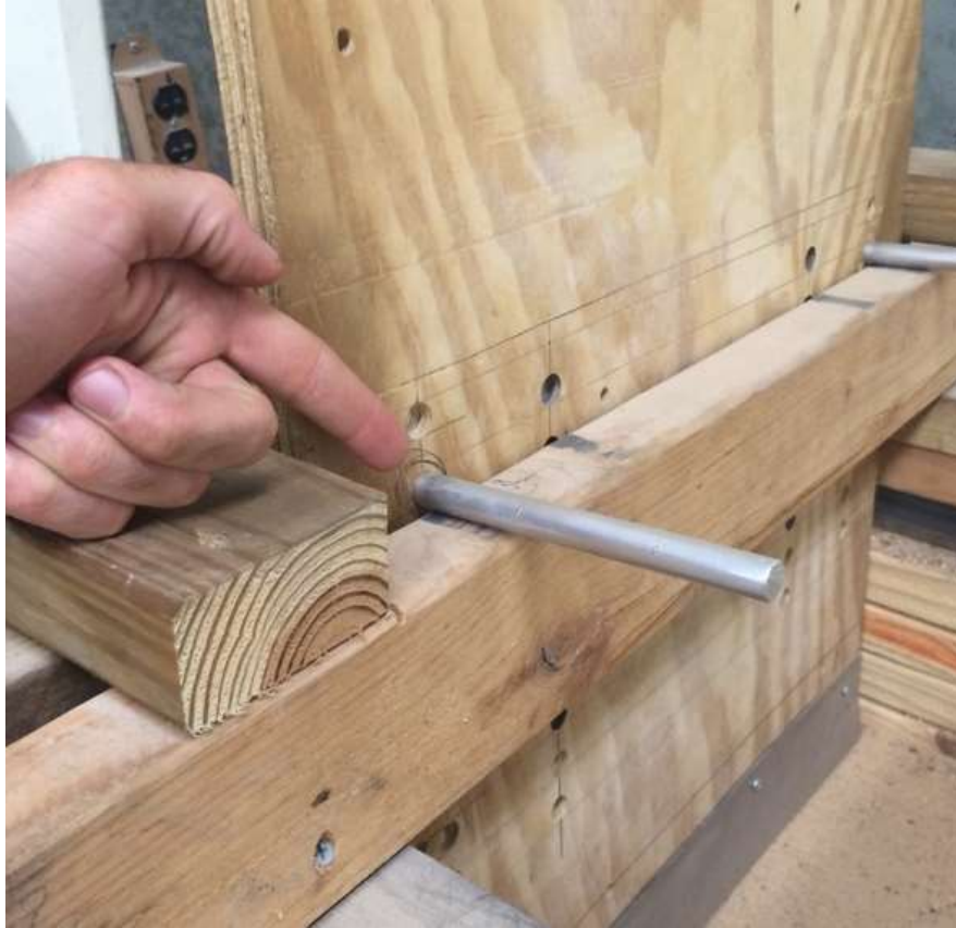
Figure 59: Aluminum rod fitted into a hole drilled in the plywood plate
