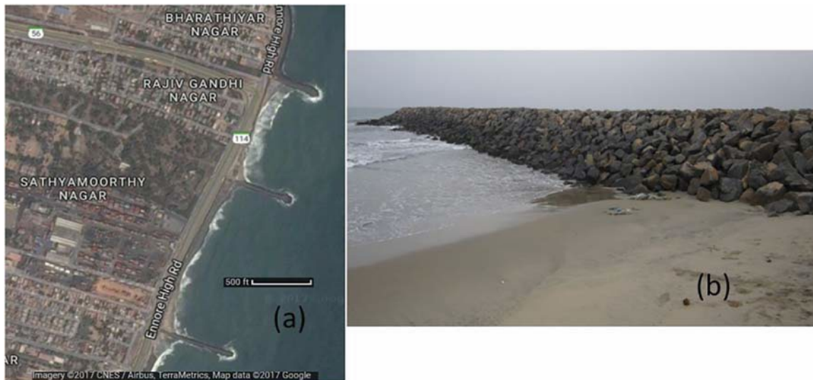
Figure 5.2 (a) The groins installed along North Chennai beaches; (b) a close-up view of a groin.
