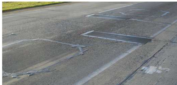
Figure 3.1: WIM Station – bending plate and inductive loops. (Hallenbeck, M. and Weinblatt, H. 2004)
