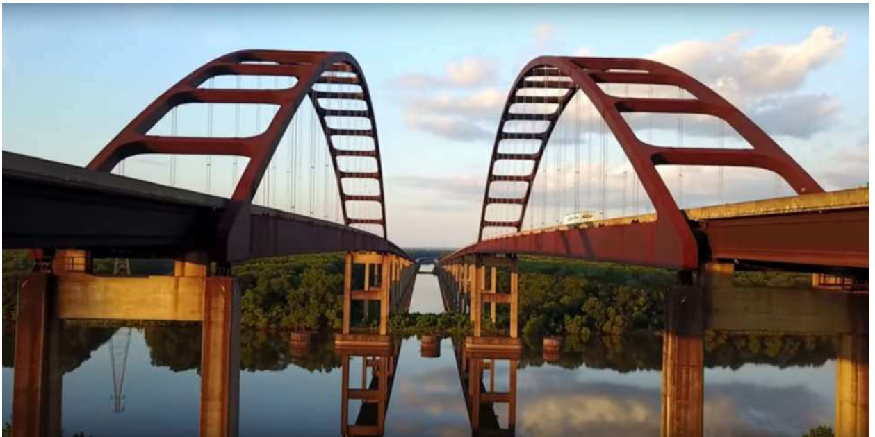
Figure 5.1: Overview of the General W.K. Wilson Jr. Bridge ( https://www.youtube.com/watch?v=LjtkE5WLjys ).
