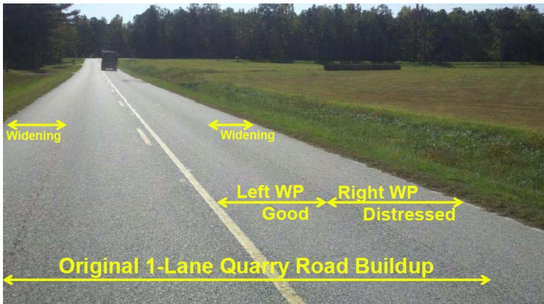
FIGURE 4.10 Condition of the low volume road section.
