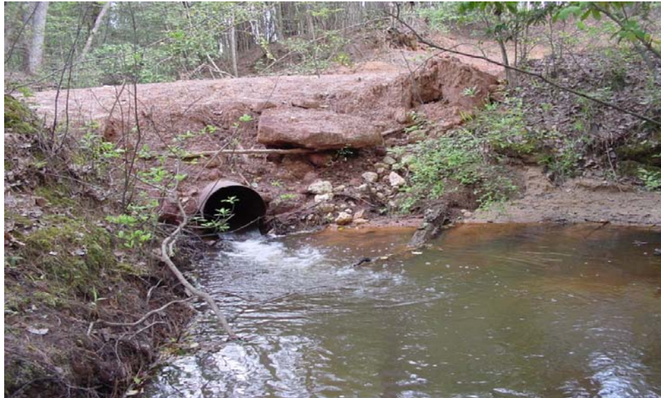
Figure 2.10 Road stream crossing constructed after harvest on 8 Dec, 2004. Refer Figure 2.1 for location. (Source: Texas Forest Service)
