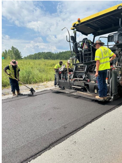
Figure 28. Material Immediately After Placement
