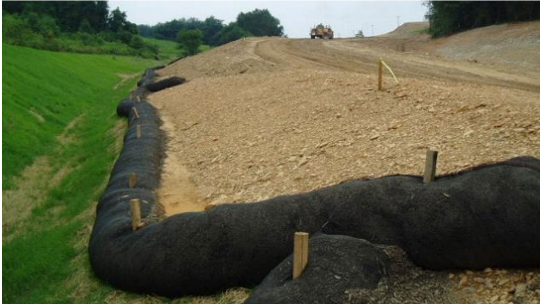
Figure 3.4: Compost Sock Installed as Perimeter Control (Perez 2016)
