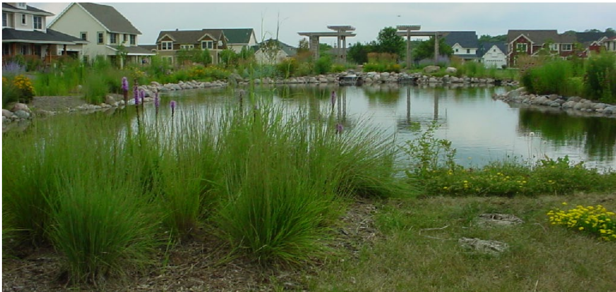
Figure 2.2: Wet Pond SCM (MnDOT 2024)
