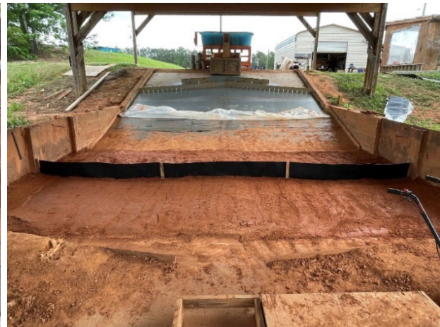
(b) view from downstream
