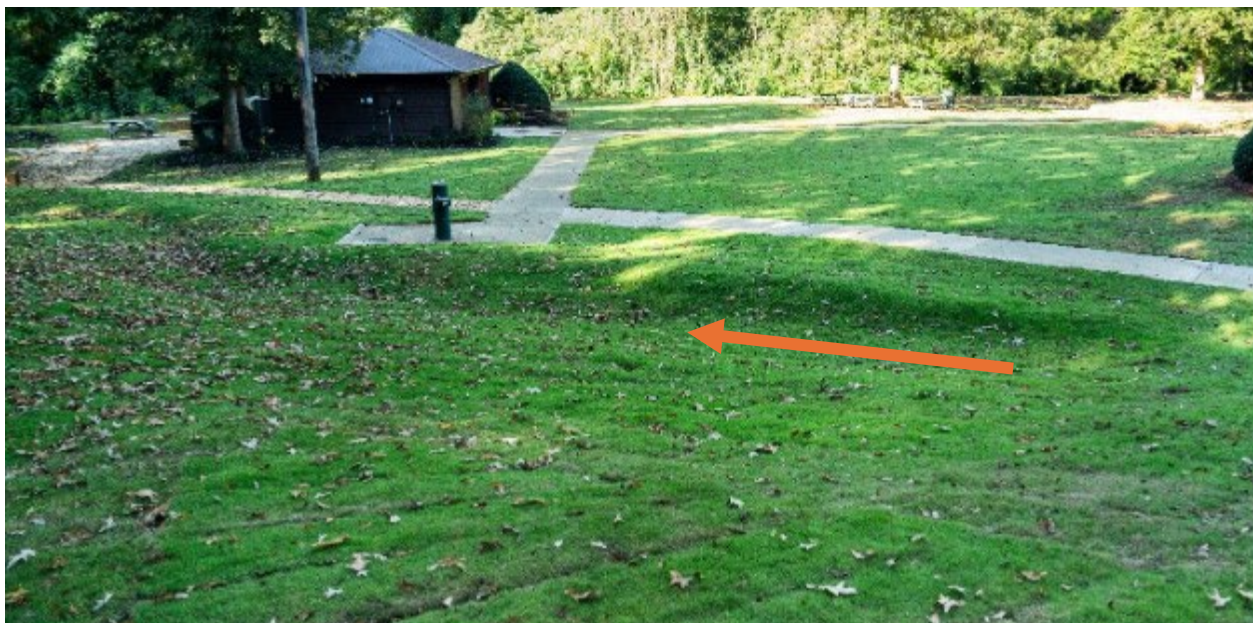
Figure 2.3: Vegetated Swale at Hickory Dickory Park, Auburn, AL
