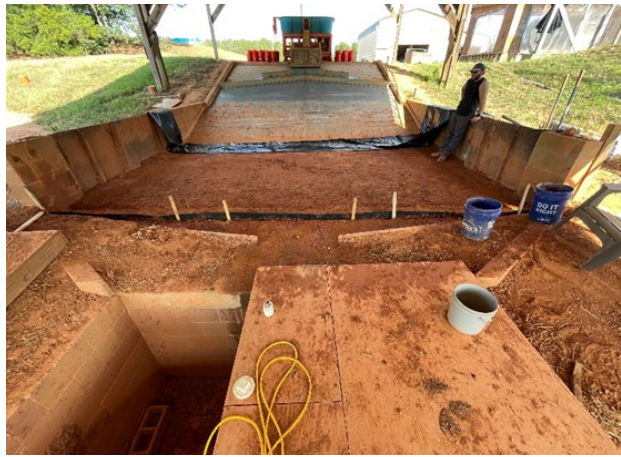
(b) view from downstream
