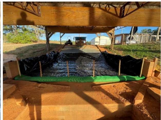
(b) view from downstream
