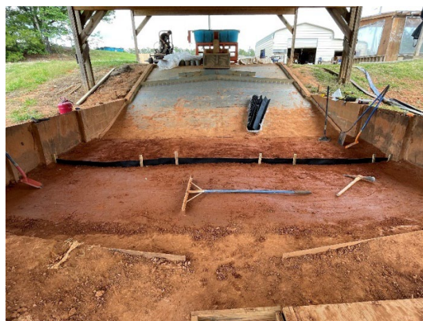
(b) view from downstream
