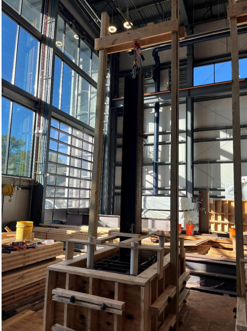
Figure 87. Support frame for steel H-piles. Specimen ready for casting.
