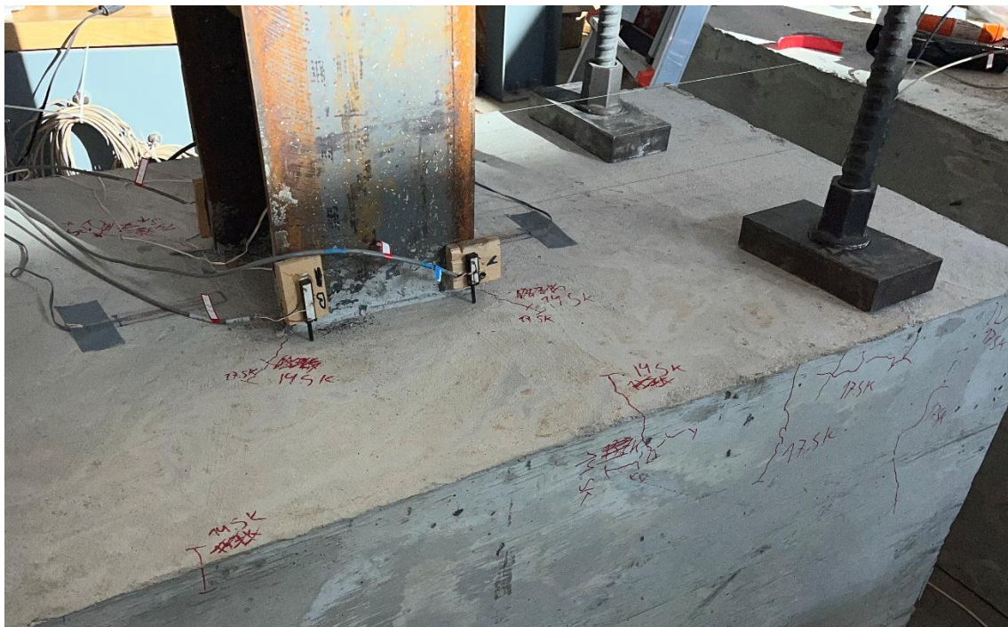
Figure 104. Specimen W-10-15 crack formation after target loads of 14.5 kips and 17.5 kips (applied loads of 13.8 kips and 15.8 kips, respectively) (load direction: from right to left).
