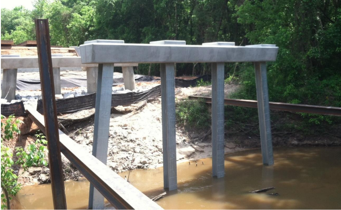
Figure 61. Typical Pile Bent with Galvanized Steel HP Piles and Reinforced Concrete Cap (Marshall et al, 2017).
