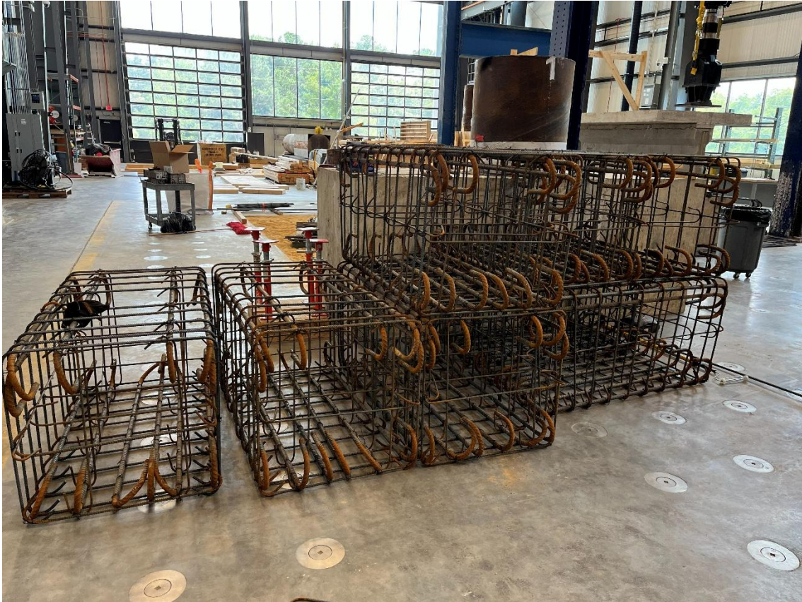
Figure 84. Reinforcement cages ready for placement.
