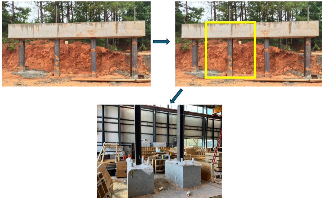
Figure 78. Experiment Conceptualization of a single specimen of a concrete bent cap with a steel H-pile.
