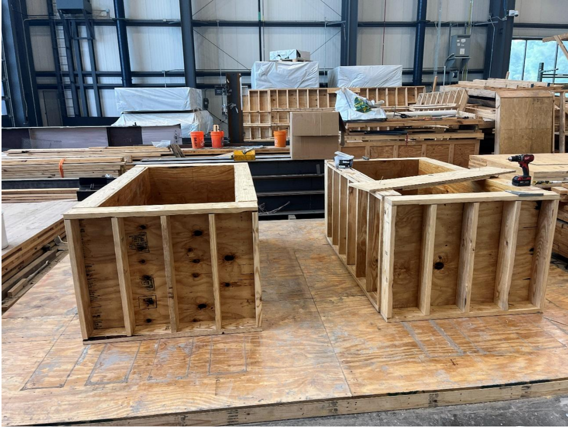
Figure 85. Formwork ready for Reinforcement cage placement.
