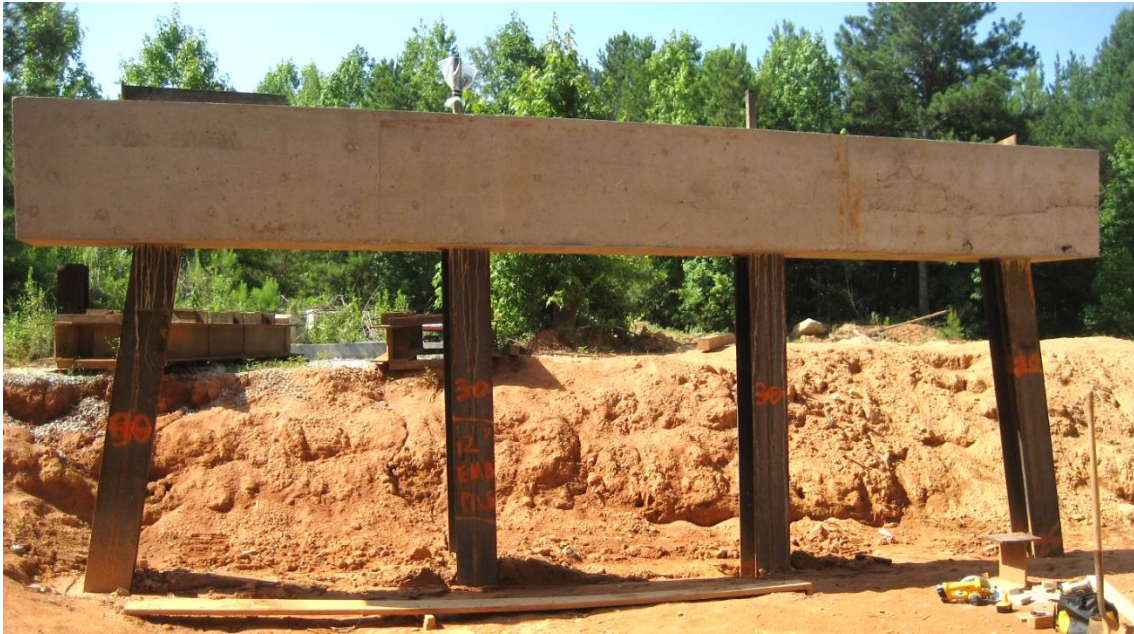
Figure 64. AUNGES battered test bent (from left to right: piles 1, 2, 3 and 4), in Lee County, Opelika, AL. Horizontal load applied from right to left. (Marshall et al, 2017).
