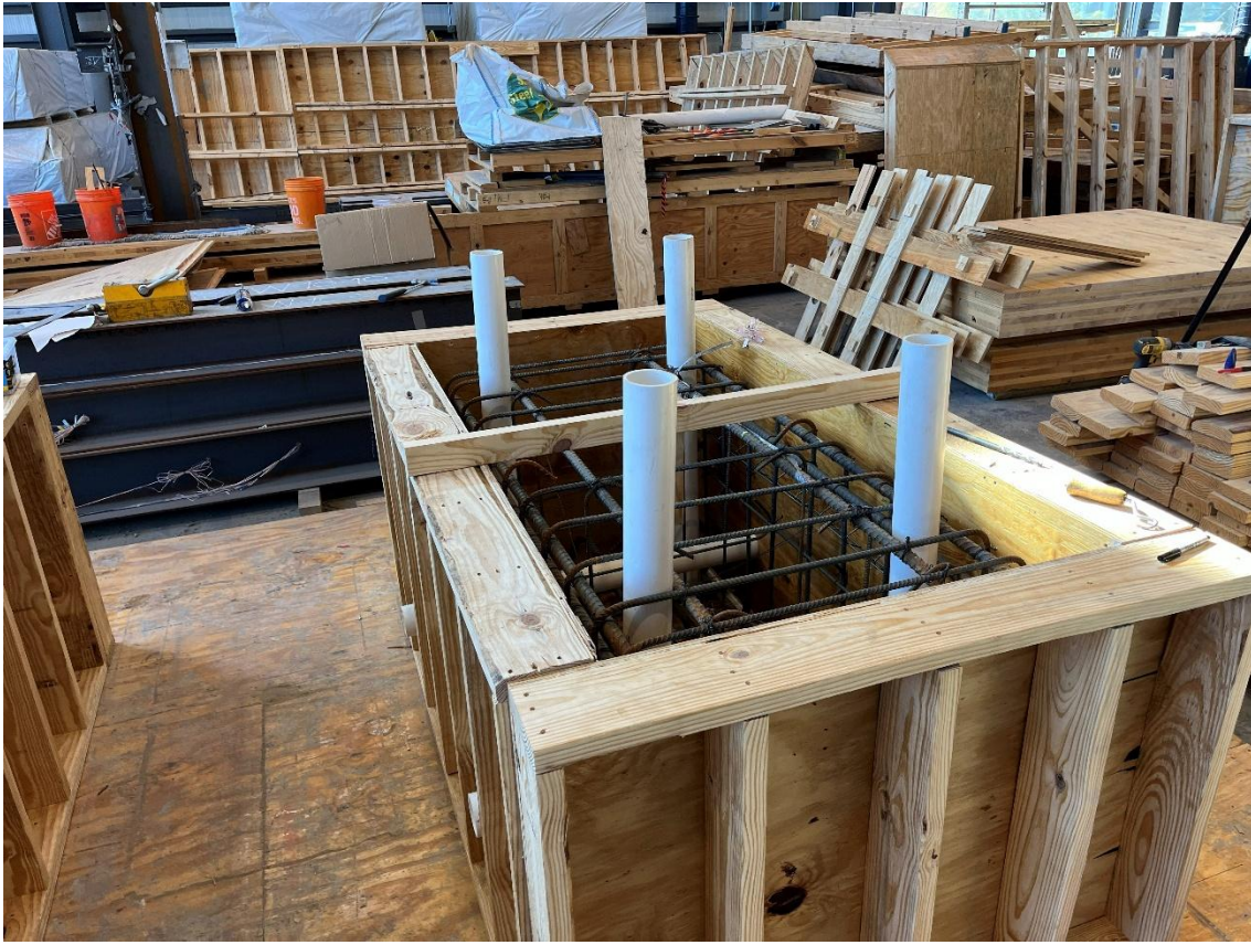
Figure 86. Formwork and reinforcing steel cage ready for pouring.
