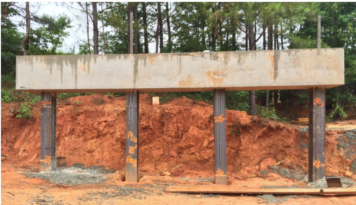
Figure 65. AUNGES vertical bent test (from left to right: piles 8, 7, 6 and 5), in Lee County, Opelika, AL. Horizontal load was applied from left to right (Marshall et al, 2017).
