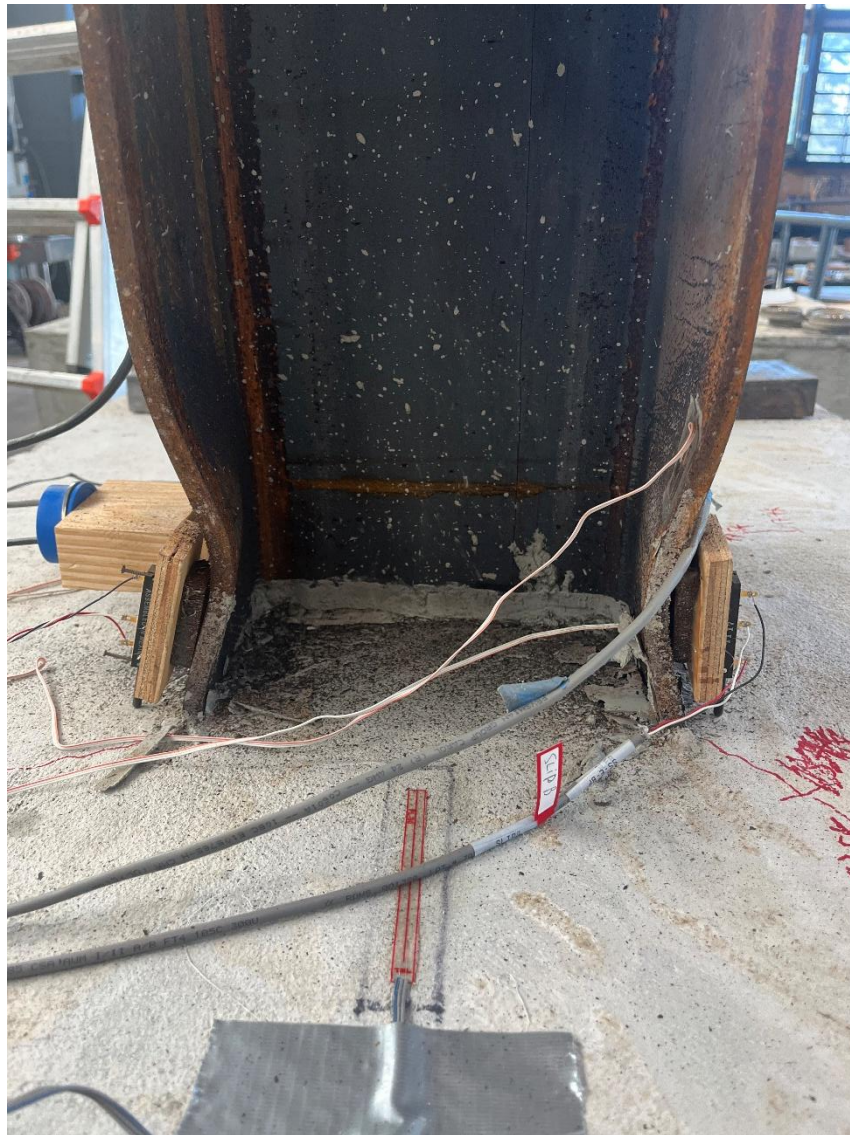
Figure 105. Specimen W-10-15 after final load stage (approx. 16 kips). Observed buckling in flanges B and C and mill scale loss.
