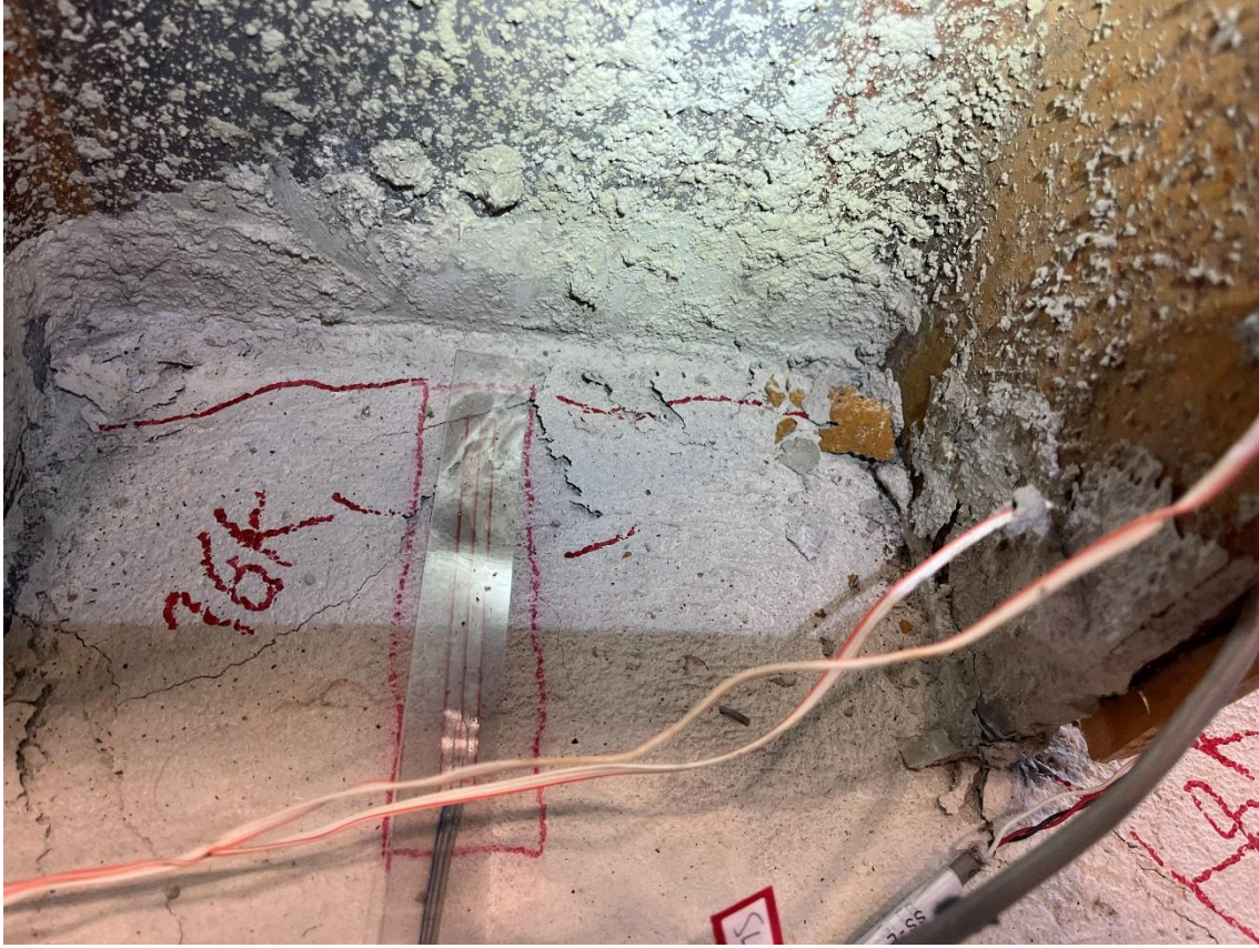
Figure 129. Specimen W-10-7.5R after final load stage (target load 16 kips, actual load 8.7 kips). Observed excessive concrete crushing on the leading side.
