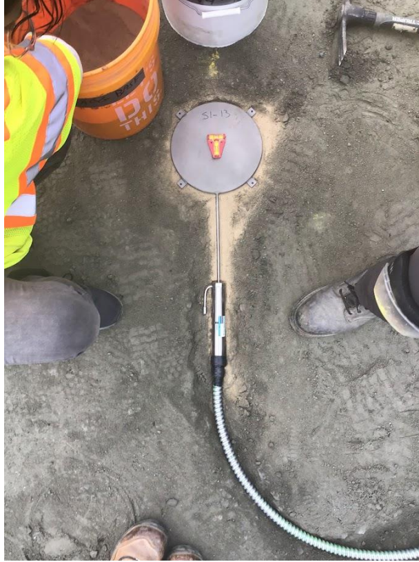
Figure 3.7: EPC Placement Before Paving
