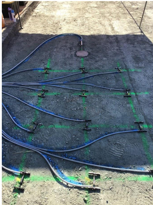
Figure 3.6: Section Gauge Array on Top of Aggregate Base
