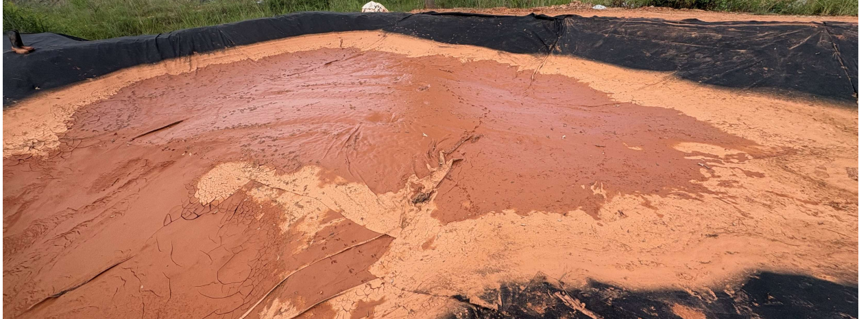
(a) Channel Upstream of Sediment Trap
