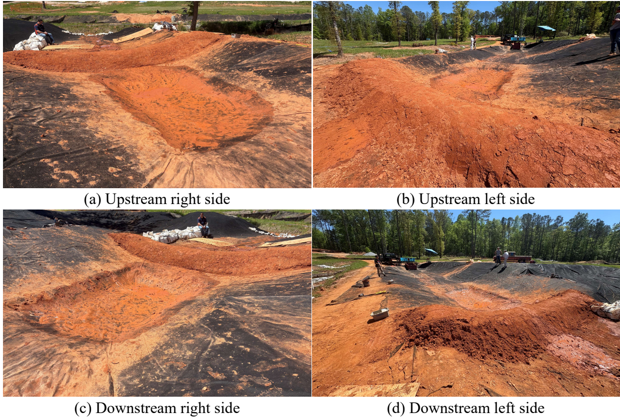
Figure 4.9: Temporary Earth Check
