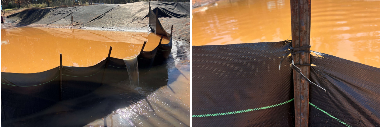
(a) Installation behavior
