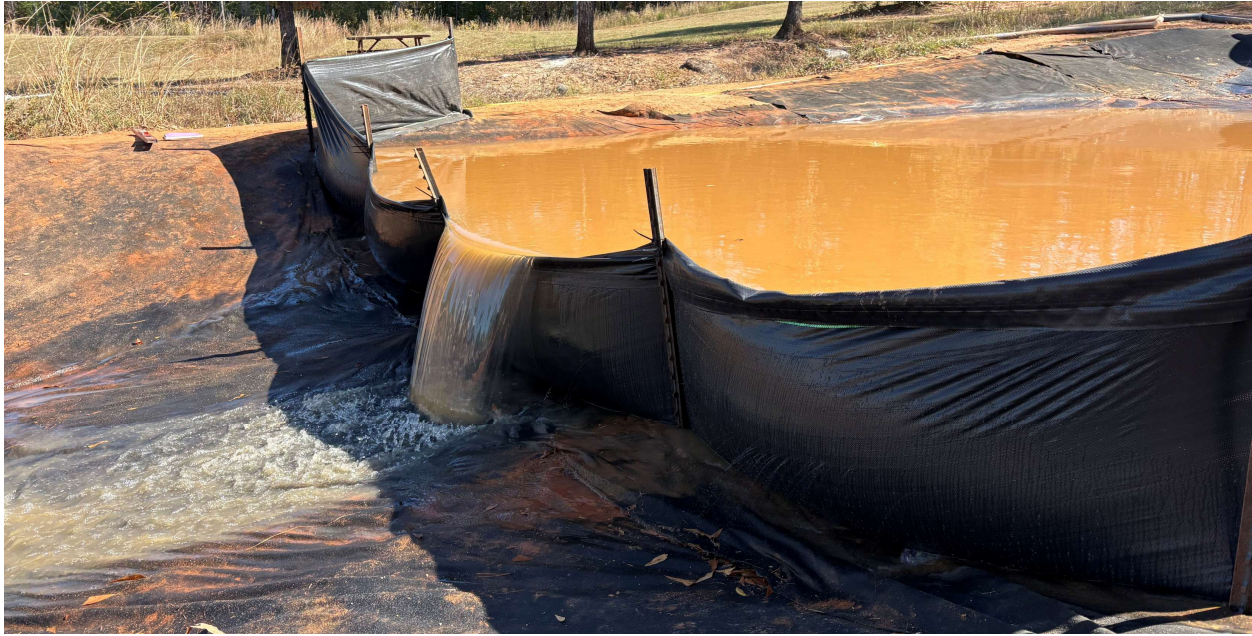
Figure 4.21: Installation 1 After Test C
