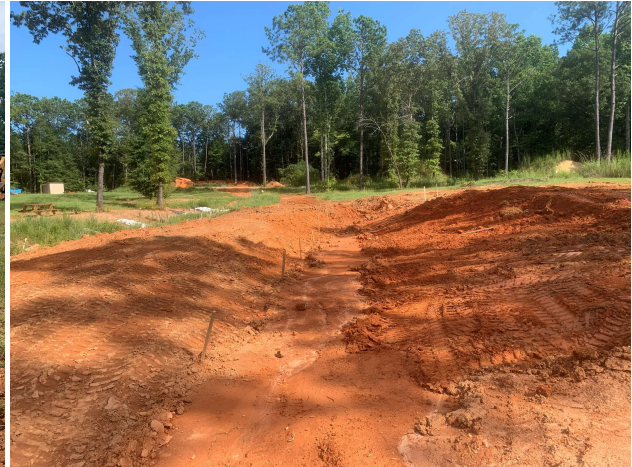
(b) Rough Grading Stage
