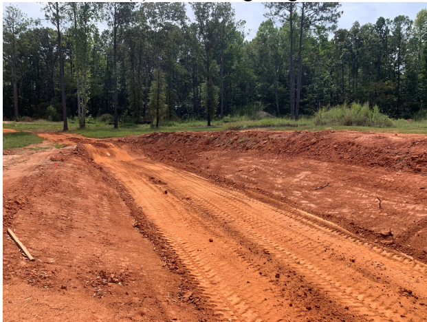
(c) Fine Grading Stage
