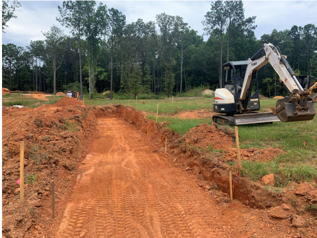
(a) Excavating Stage
