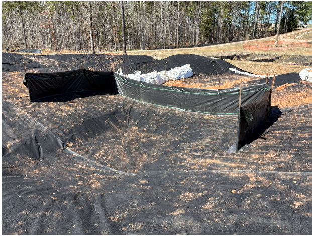
(a) Standard low porosity silt fence
