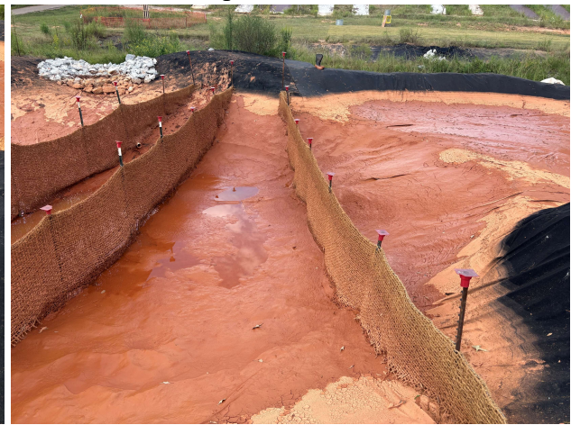
(c) Second Bay of Sediment Trap
