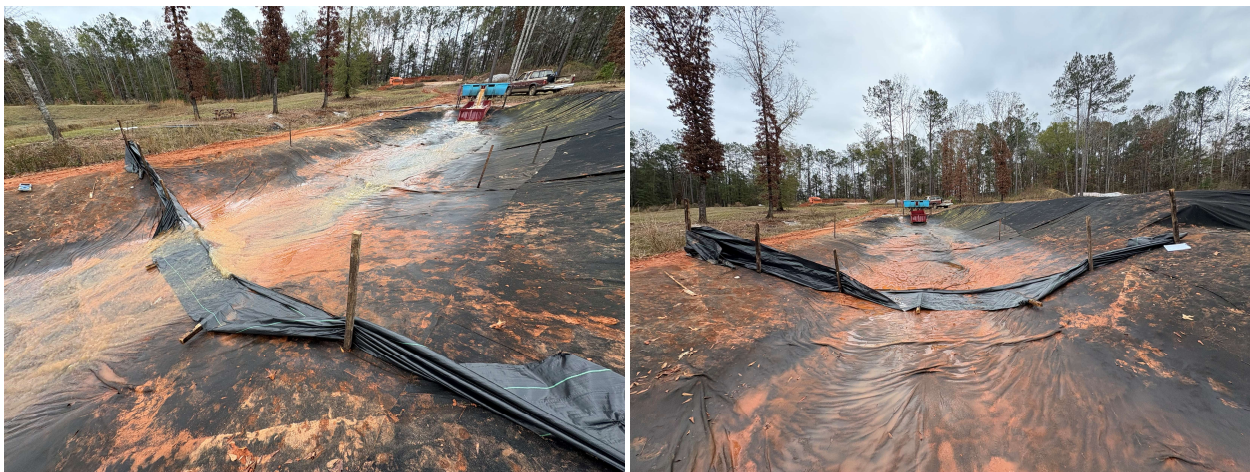
Figure 4.26: Installation 4 Failure
